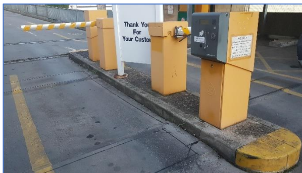
Level 9 barrier access to Rock Road
